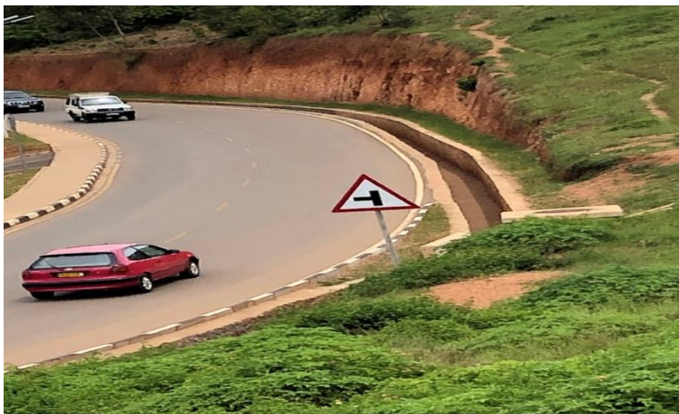
Figure 27: Drainage structures beneath the proposed campus site
