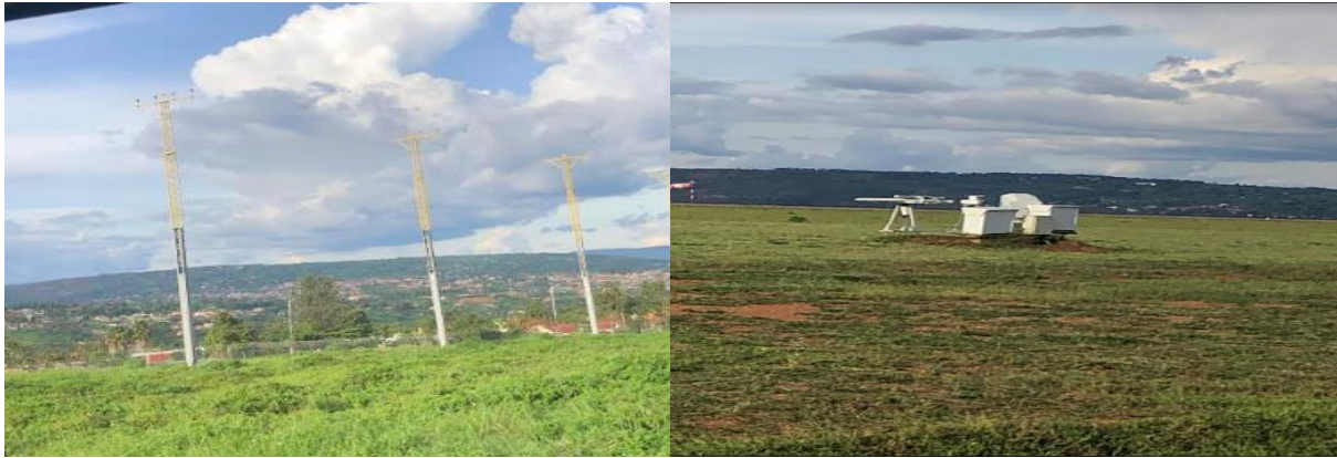
Figure 1: Some of the utilities existing at the KIA.
