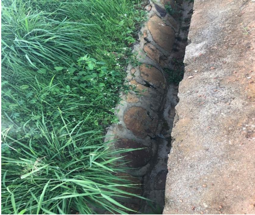
Figure 23: Drainage structures next to the aircraft hangar site
