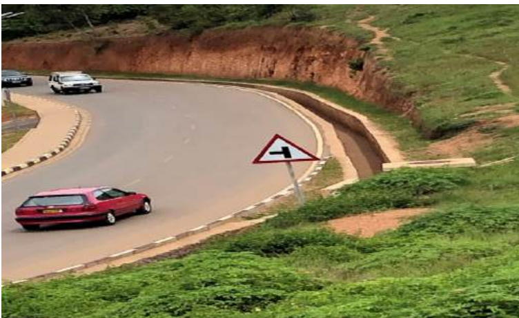
Figure 27: Drainage structures beneath the proposed campus site
