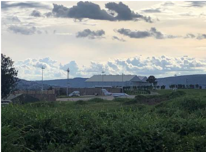
Figure 24: Existing apron next to the aircraft hangar site
