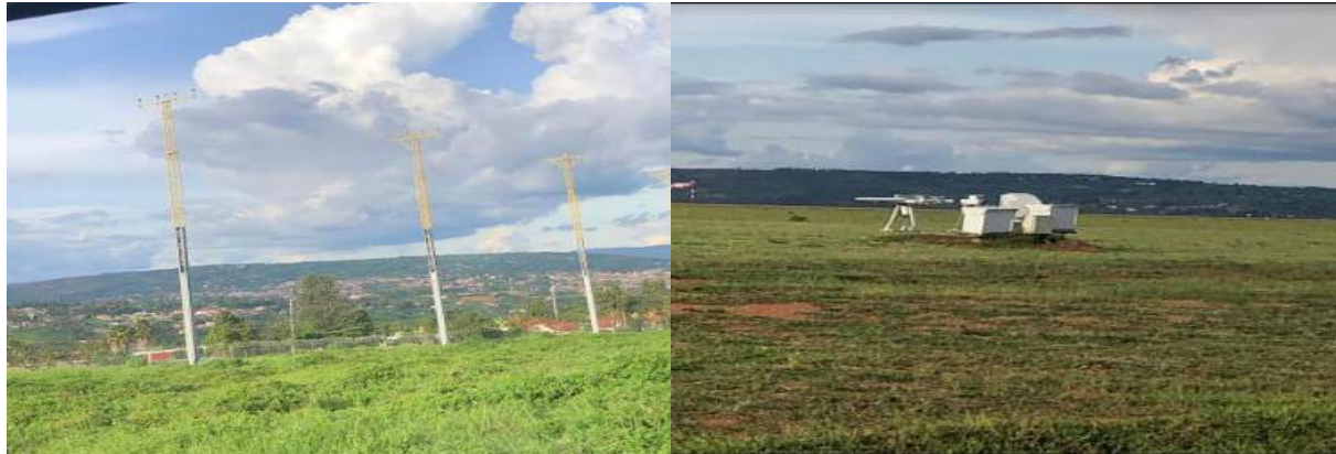
Figure 1: Some of the utilities existing at the KIA.
