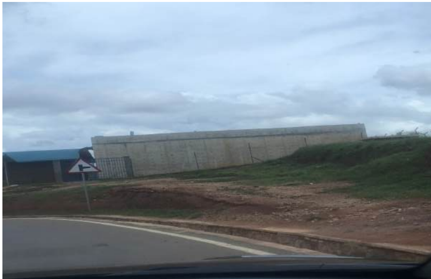
Figure 33: WASAC water tank next to the proposed aircraft hangar site.
